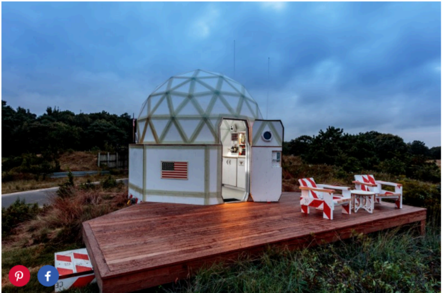
An exterior view of Building #3 .
